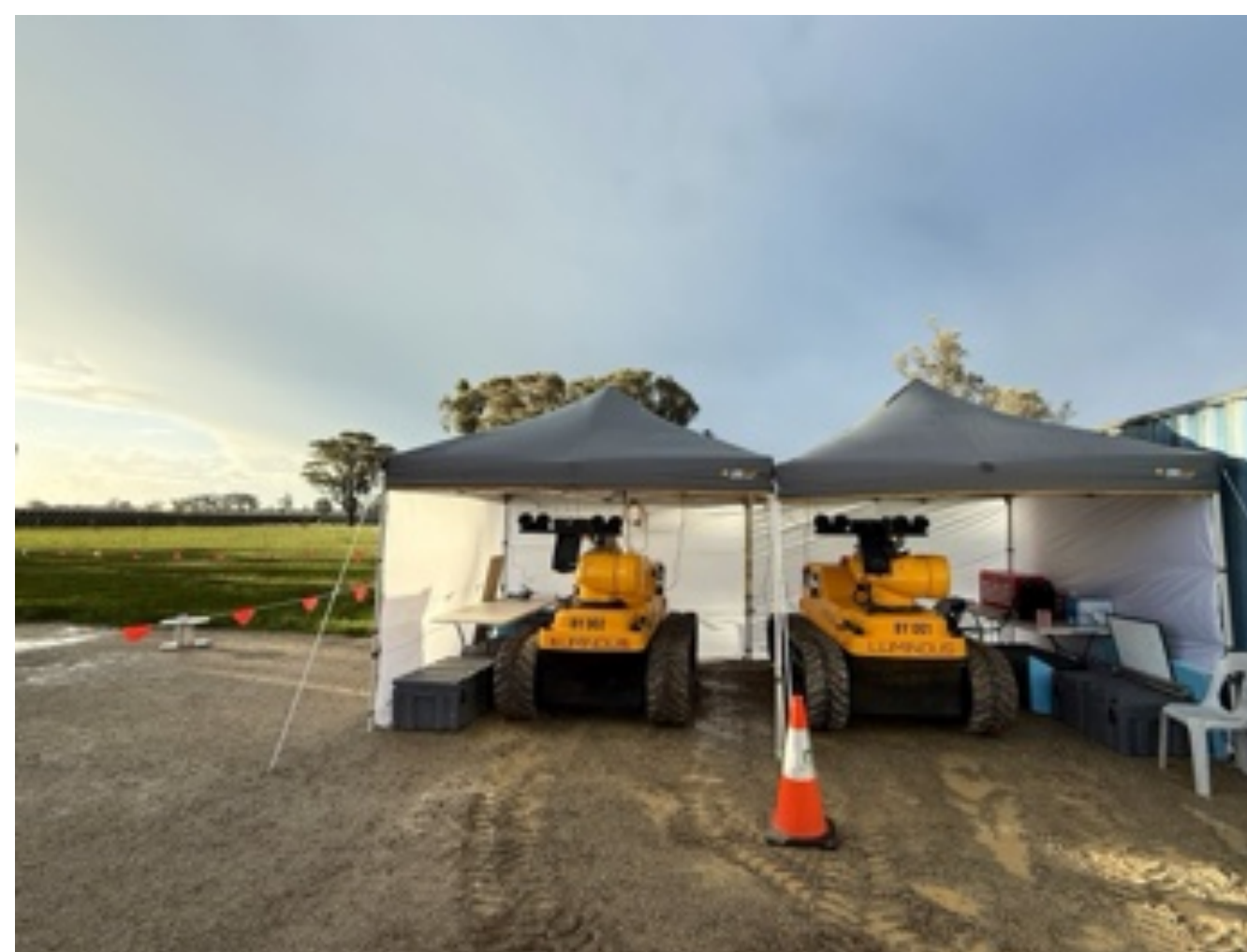
Goorambat East Solar Farm //
