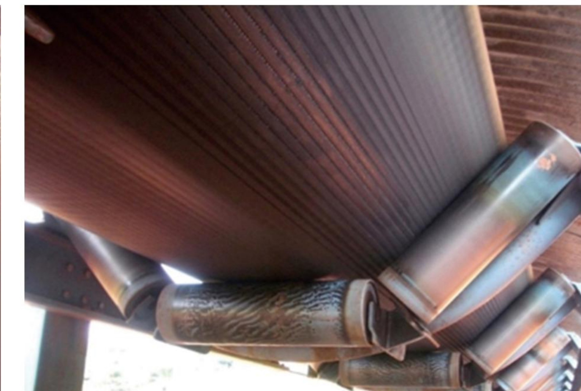
Belt cover wear due to forward tilt of idler
