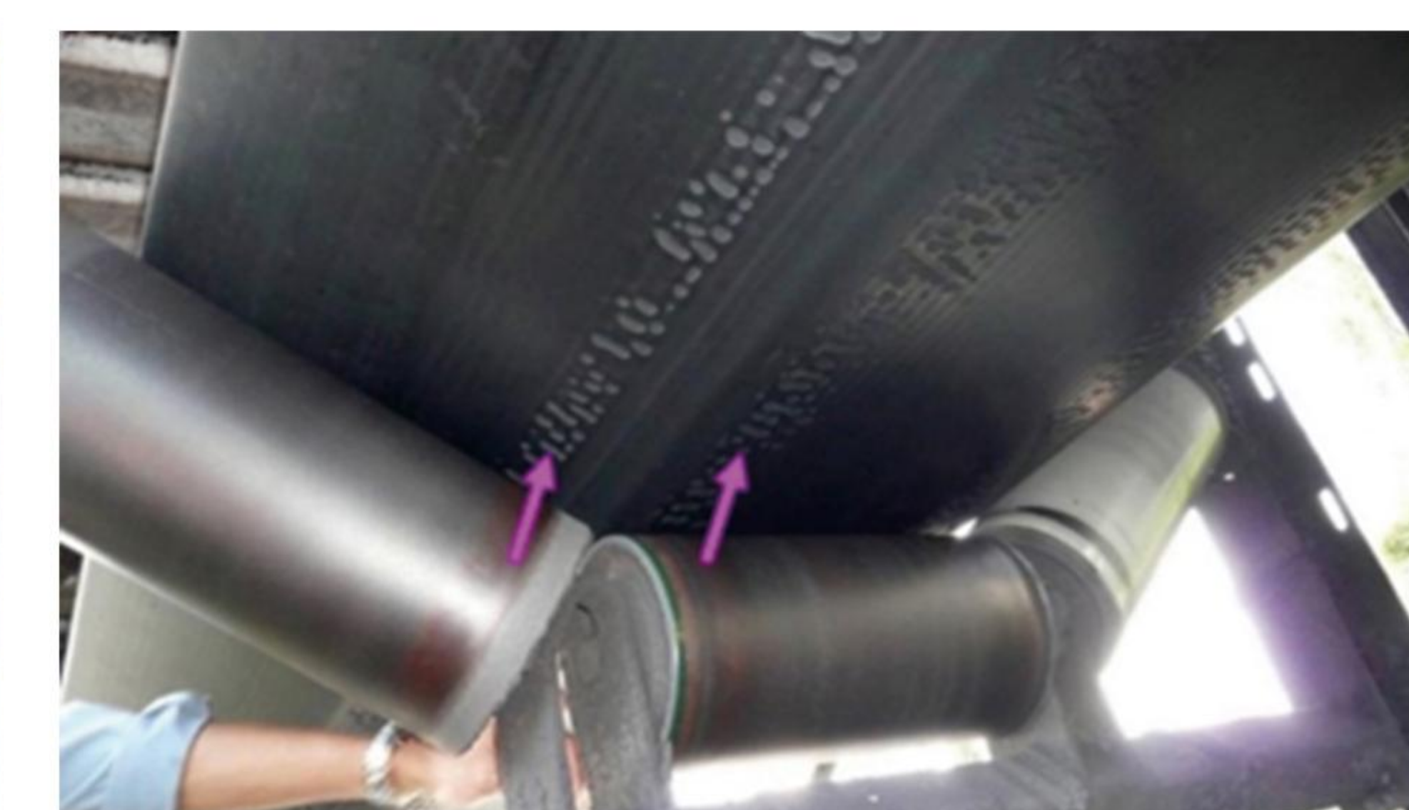
Underside damage in high contact pressure area
